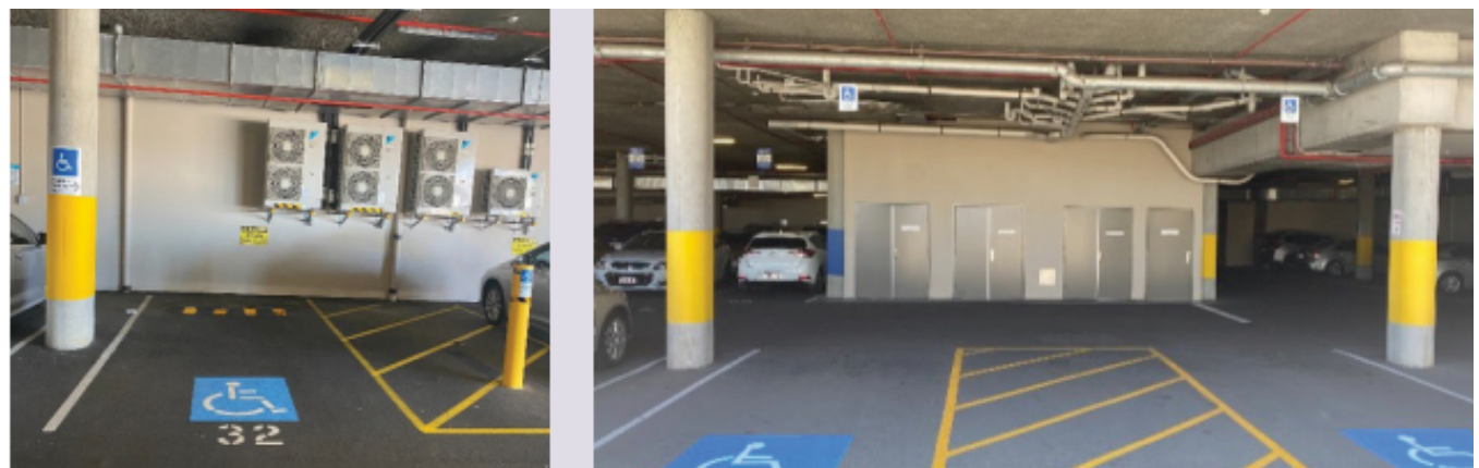
Underground ACROD parking bays off Yagan Place. Lift located in car park.
