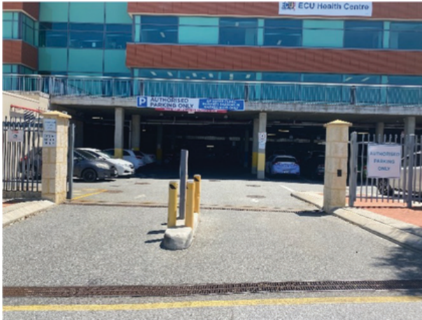
Entrance to underground car park off Yagan Place.
